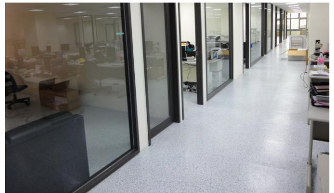
office renovation project, top-finish by vinyl tiles
